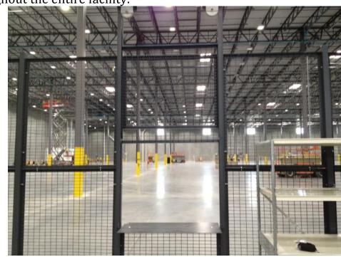
move up and down gradually in a safe manner. Each service window has a padlock lug so the window can be locked in the opened or closed position.
